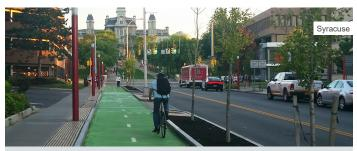
**Separated Bike Lanes (SBL)**—similar to standard bike lanes, SBLs include a buffer with a visual or physical barrier between moving cars and bicyclists. Barrier options include flex posts, a row of parked cars, or a narrow landscaped median (as shown). SBLs can be located on each side of the street or as a bi-directional facility.
